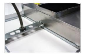
The MAC 10<sup>®</sup> LEDC 4x4 maximizes energy efficiencies with its exclusive backward blower wheel design. It provides 90 fpm airflow up to 1.0" wg static pressure levels enabling cleanroom projects to operate cost effectively. Fewer components mean lower installed costs. With use of the MAC 10<sup>®</sup> LEDC 4x4 unit, additional savings are captured in the ceiling plenum because less grid is required and fewer electrical connections are needed.
